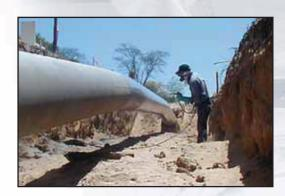
All Powercrete® formulations are developed to be field friendly and cost effective. The ease of application can be achieved either by hand (rollers, brushes or trowels) or with spray equipment which delivers high-build in a single pass, thereby reducing application time. This engineered application flexibility allows the contractor to stock and manage a single product for any application requirement.
