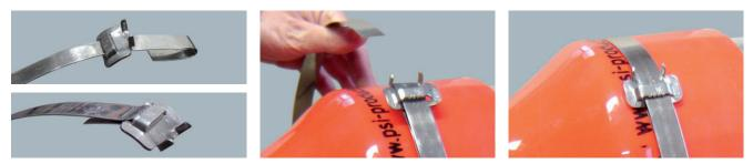
1. Push the stainless steel loop onto the strap; make sure that the barbs point to the end of the strap. Bend over the end of the strap about 3 to 4 cm and strike it with a hammer. Then place the strap around the sleeve and pull it through the loop.
