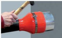
**2.** Install the first strap about 15mm in front of the end of the casing pipe.
